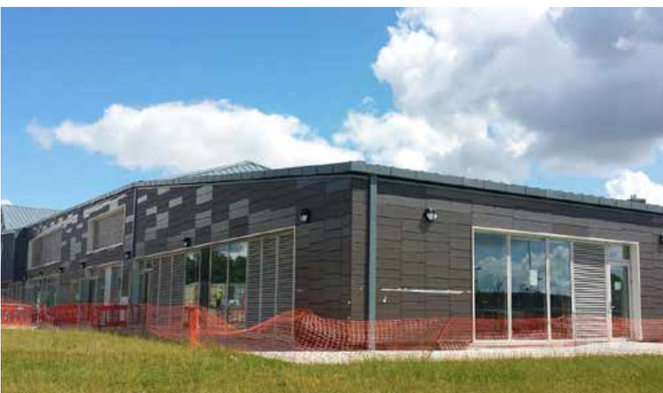
Springfield Community Campus in Corsham during construction
